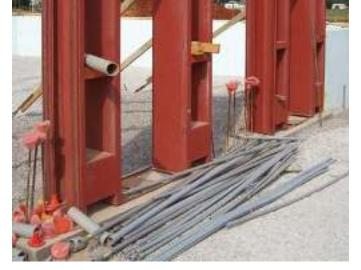
Door IFAs can be set into the floor slab, providing a mechanical connection between it and the concrete wall core.
