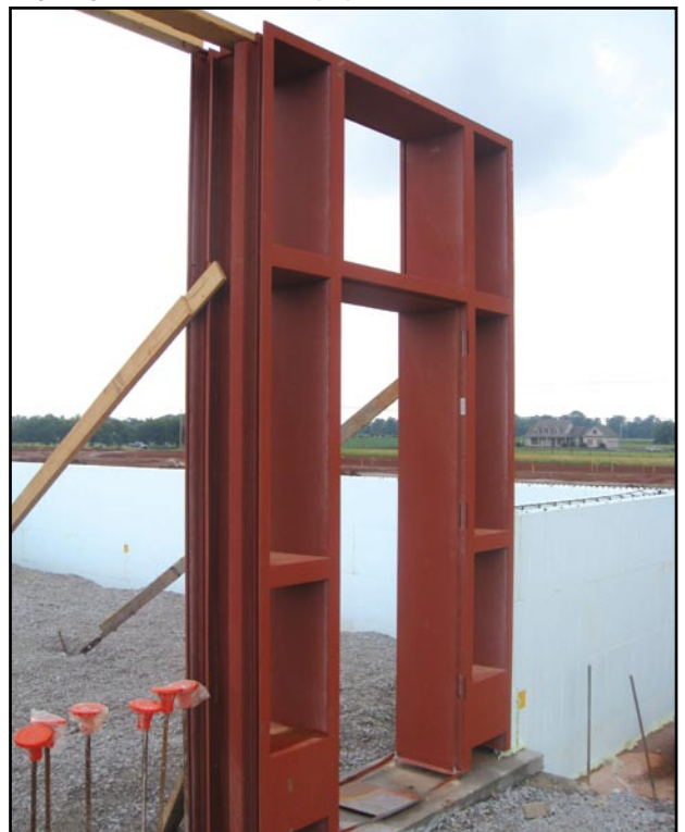
▼ Specialty IFA reflecting traditional hollow metal capabilities—including glazing, mullions, and hardware preps—anchored into footer and ICF wall.
