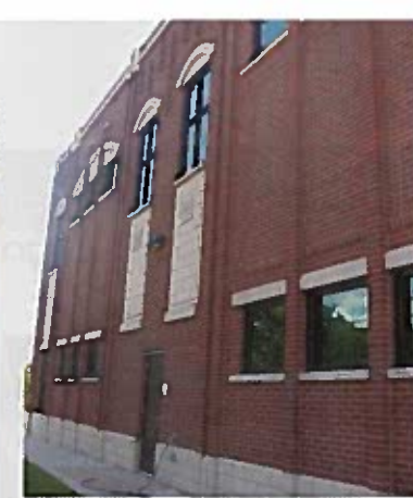
The finished exterior of the Academy, with a view of its IFA windows and door as well as one ICF wall.
