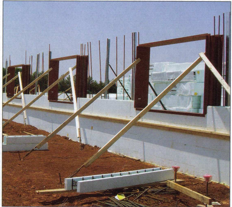
Insulating concrete forms (ICFs) offer myriad benefits, but the inclusion of door and window openings can slow building schedules. The use of proprietary integrated framing assemblies (IFAs) can prove invaluable.
