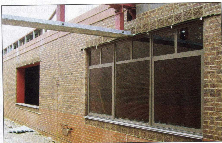
In Franklin County, Kentucky, this new elementary school relied on integrated framing assemblies for both doors and windows.
