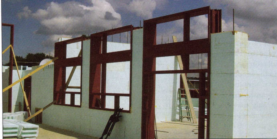
In designing the new Overdale Elementary School as an ICF project, K. Norman Berry and Associates also specified IFAs for mechanical chases. These IFAs have sidelites and mullions.
